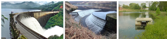
Figure 15: Photos of a reservoir, dam and a pond with hydraulic structures as flow controls
